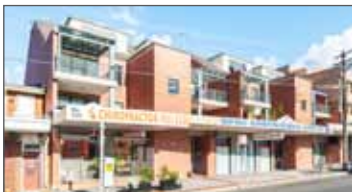
40/518-520 Bunnerong Road, Matraville
