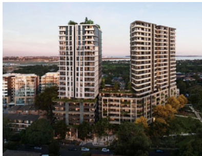
Arncliffe Central/161-173 Princes Highway, Arncliffe
