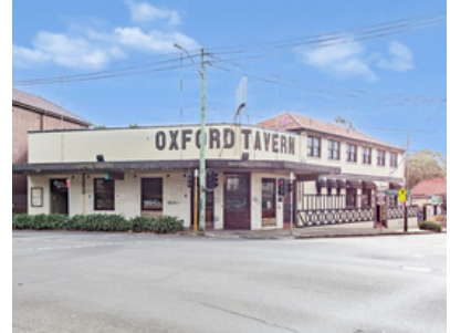
1 New Canterbury Road, Petersham
