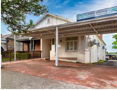
161 First Avenue, Five Dock
