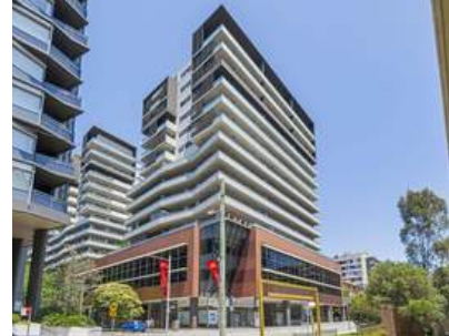
Suite 9, Level 2, 1-17 Elsie Street, Burwood
