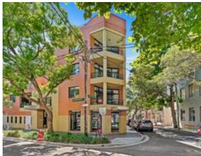
Shop/18-20 Buckland Street, Chippendale
