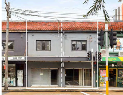
240-242 Liverpool Road, Enfield
