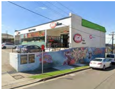
190-194 Liverpool Road, Enfield
