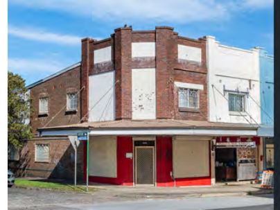
466 New Canterbury Road, Dulwich Hill
